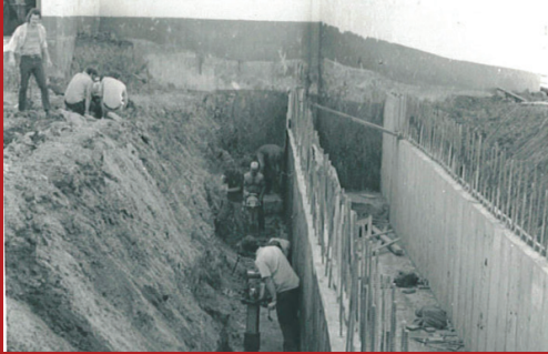
Building the Baileyville, KS grain elevator in 1961
