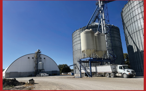
NOW: Trucks unloading at the new Wamego Grain Storage & Bin facilities.
