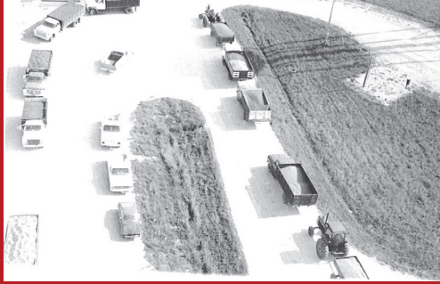
THEN: Trucks unloading at the Seneca Bunker facility.
