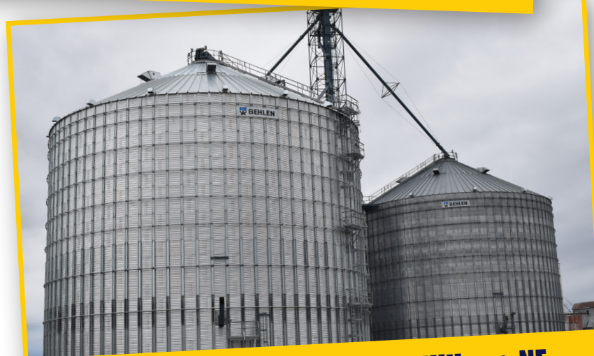
New 400,000 Bushel Bin in Milligan, NE
