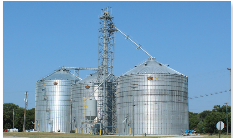
This newly-constructed bin in Ohio will be a great asset this harvest
