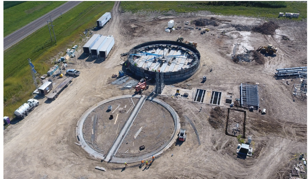
Construction continues on greenfield site near Barnes, KS.
