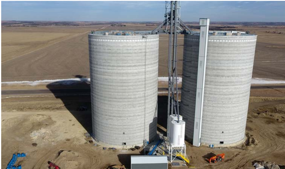
Construction nears end on greenfield site near Barnes, KS.
