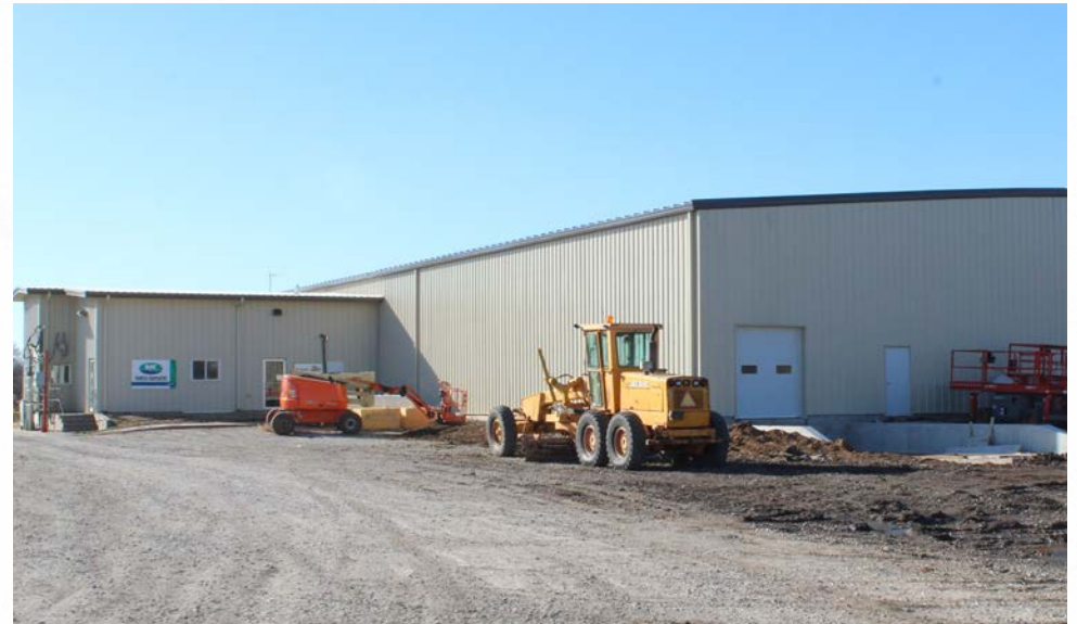
Construction progress at Wilber agronomy building.
