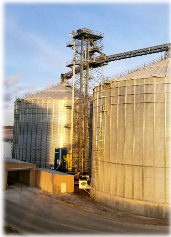
New 850,000 bushel storage facility and new 20,000 bushel per hour receiving facility.
