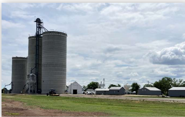
Midway Coop's newly acquired Lucas elevator facility in Lucas, Kansas.
