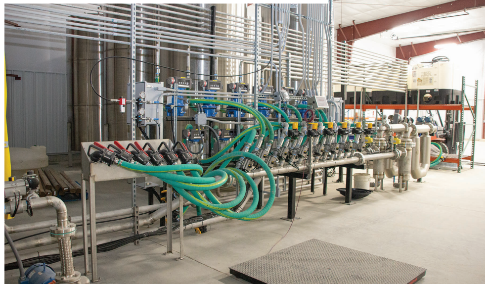
The newly constructed facility provides agronomy inputs to area growers.
