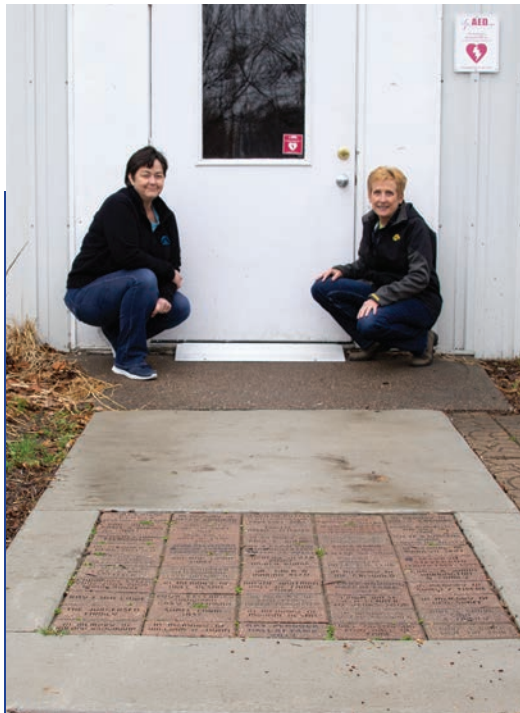
Mary Stevenson, Clinton County Agricultural Society Secretary, and Cheryl Paasch, mother of Joshua, Dawn (Vander Heiden) and the late Jason Paasch next to the sidewalk that was installed, making the Clinton County Fairgrounds more handicap accessible.
