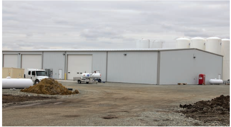
Construction is underway in Camp Grove, Illinois.
