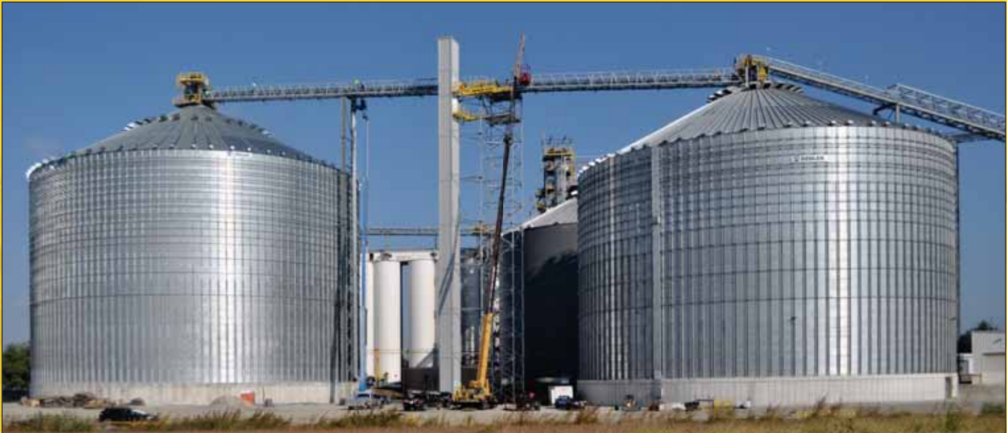
Ground-level view of two of the newer Behlen tanks built at South Charleston, including a 2-million-bushel tank at left from 2021 and a 1-million-bushel tank from 2020 at right. Ground-level photos by Ed Zdrojewski.
