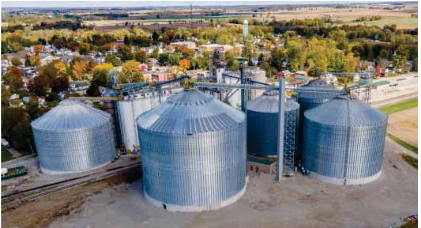
The new Behlen 2-million-bushel tank at Sunrise Cooperative rail terminal in South Charleston, OH is the largest corrugated steel tank the manufacturer has built to date. Drone photo by Raines Photography, Wapakoneta, OH.
